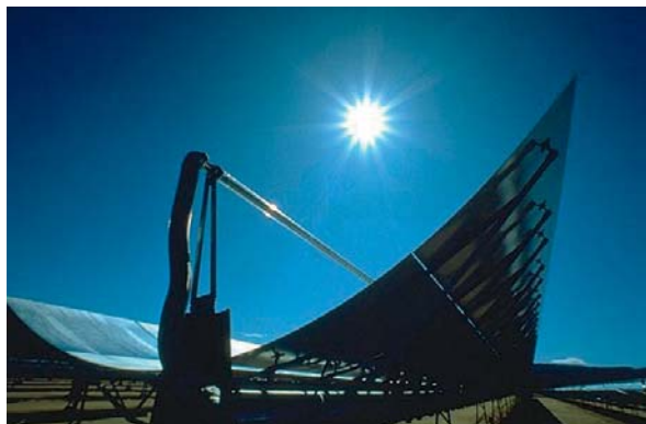
Power stations use trough shaped mirrors that concentrate the sunlight onto a pipe filled with a heat transfer medium which runs through the focal line of the mirror.
