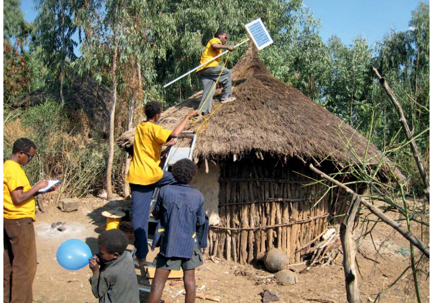
The smallest of photovoltaic facilities play an increasing role in rural energy generation. Pictured is a solar installation from the initiative, 'Licht für Bildung' (lit. 'shine a light on education') run by the German NGO 'Stiftung Solarenergie' (Source: Stiftung Solarenergie)
